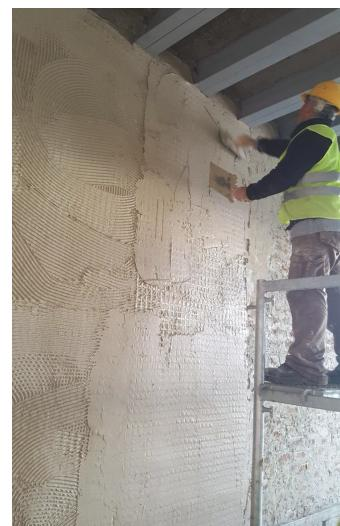
*Recent Application: Portneo is strengthening the masonry walls of two historical schools located in Istanbul using textile-reinforced mortar.*
